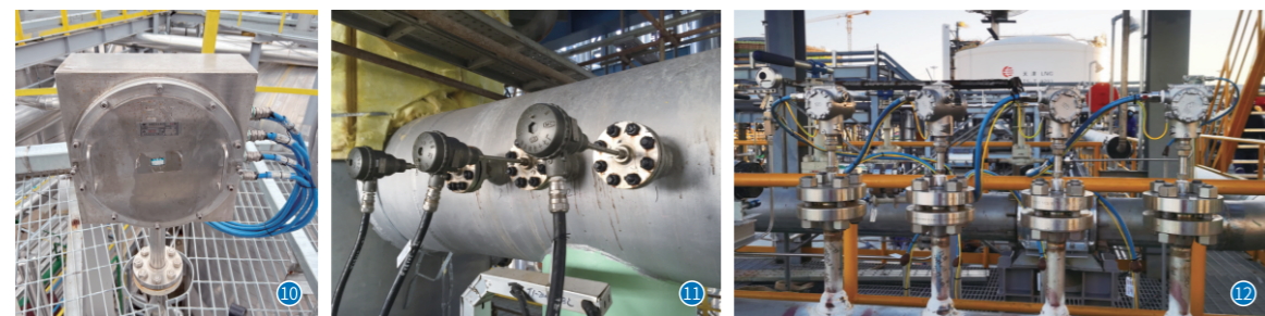
7 加热炉高精度多点热电偶 Heating Furnace TC with High Accuracy
