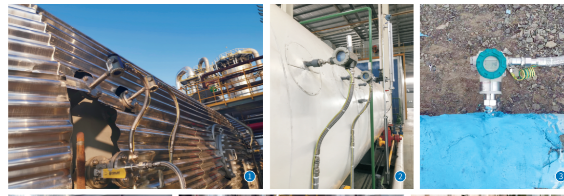
3 地面集输场站管夹式(非浸入)一体化温度变送器 Ground Gathering Station Pipe Hoop(Non-immersion) Integrated TT
