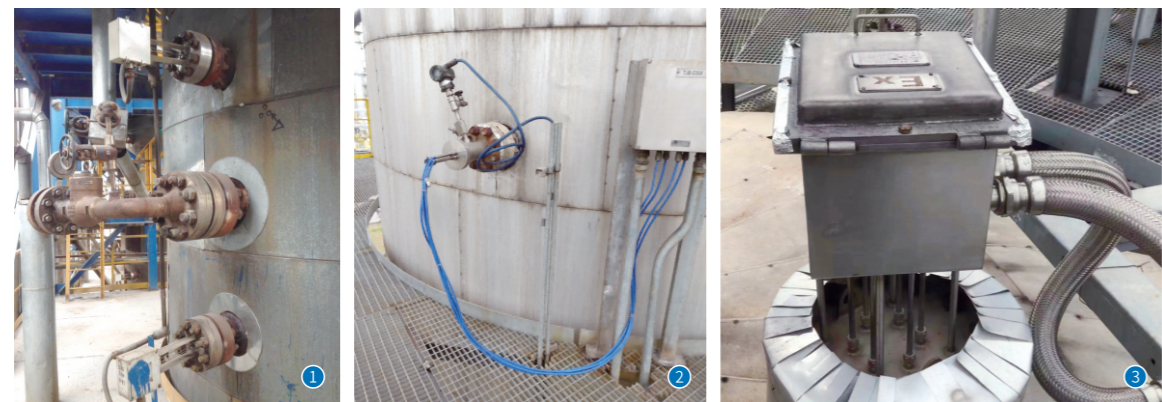
3 EO (环氧乙烷) 反应器多点热电偶 EO Reactor Multi-point TC
